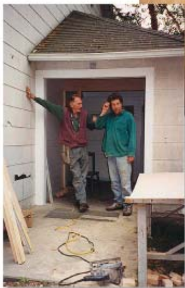
George Post, John Sumrall relocate front door of hall
